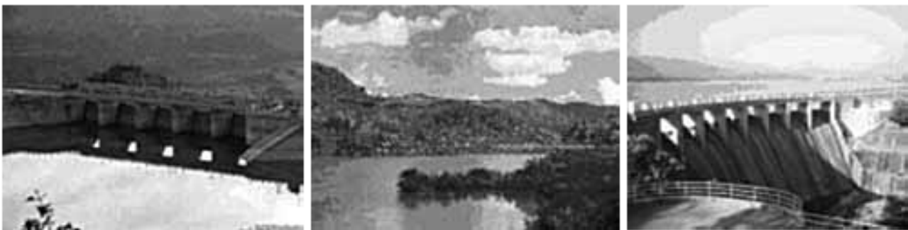
Figure 1. Dams used as a source of water supply for twin cities of Islamabad and Rawalpindi
